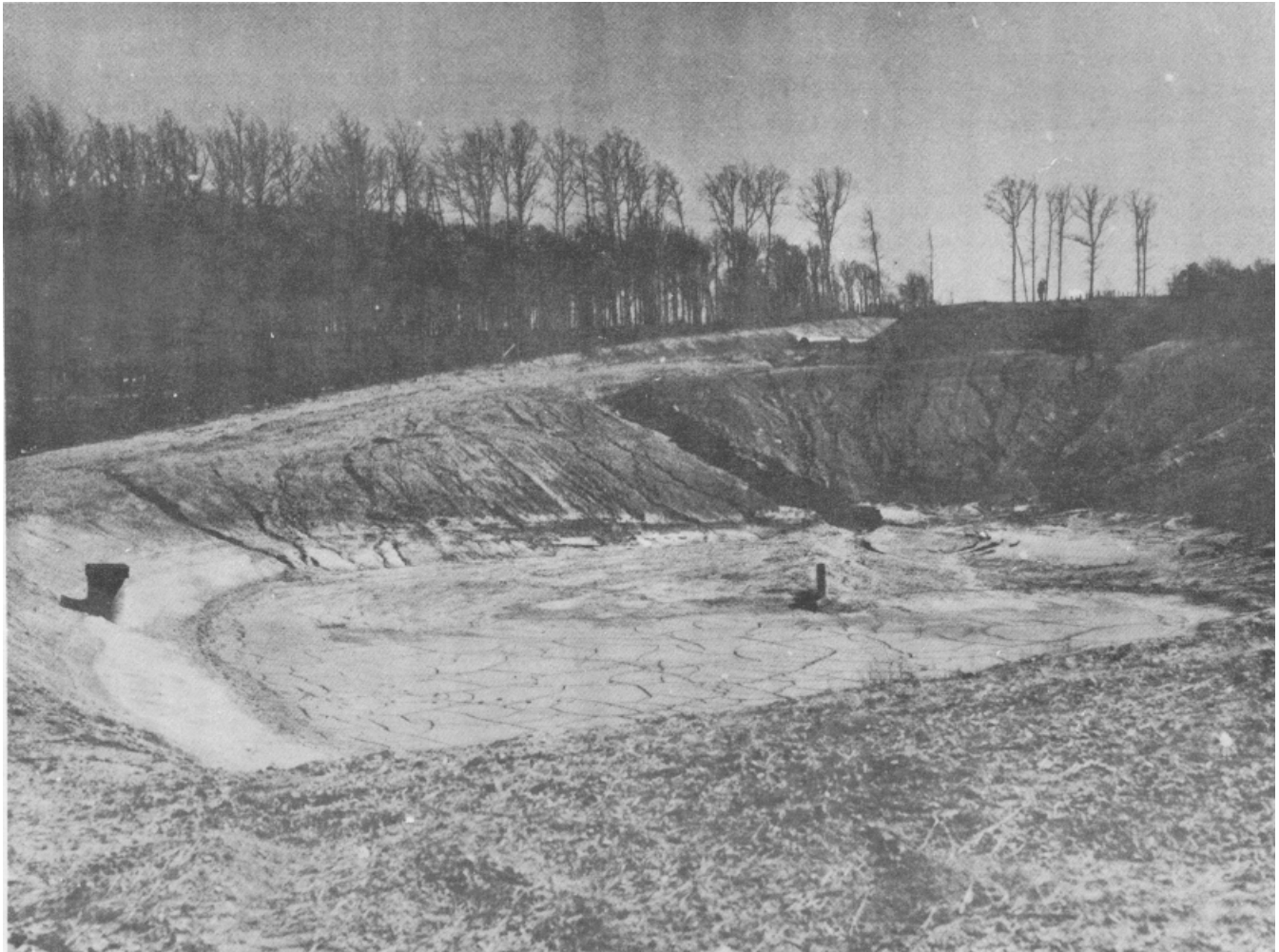
Figure 7-1. Sediment basin on a construction site.
